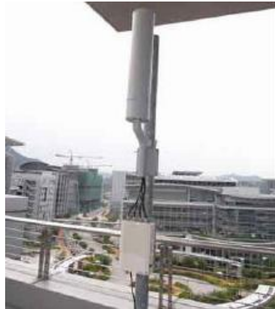
Figure 3: Altai A8T WiFi Cellular Base Station with 4-Sector Tube Antenna
